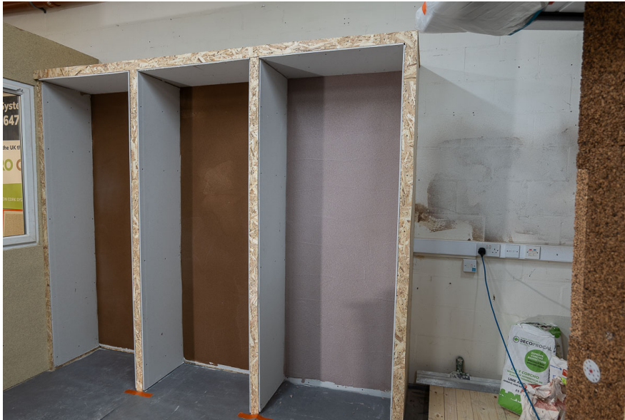
The Academy demonstration bays show the successive application and finishing stages.
