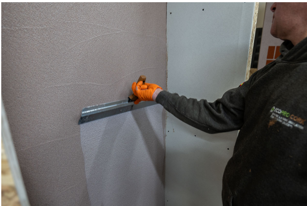
Levelling the applied material during practical training.
