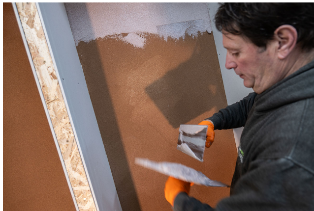
Trowel application to an Academy demonstration wall.
