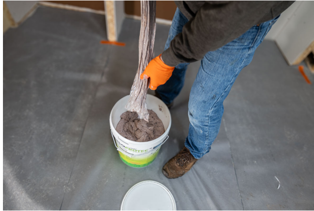
Mechanical mixing of the cork material in its bucket.
